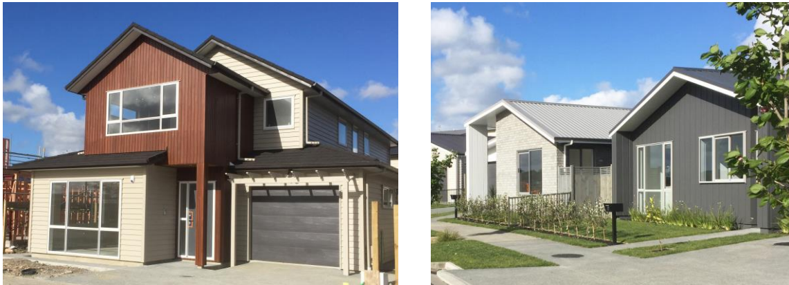
Figure 5: Examples of a variety of roof forms
